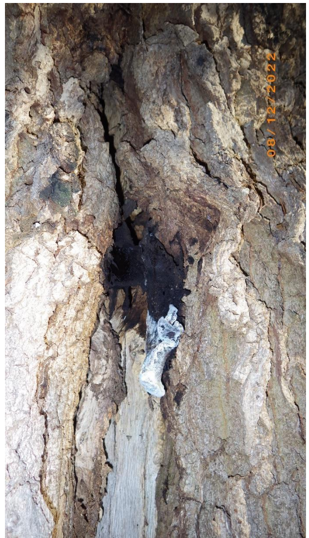
Foto 14: Baum Nr. 2 - Hohlraum in ca. 2,0 m Höhe
